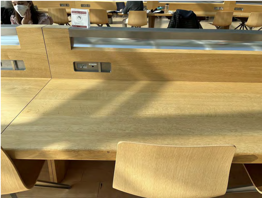
Figure 5.69 - Integrated power, data, laptop lock and lighting.
